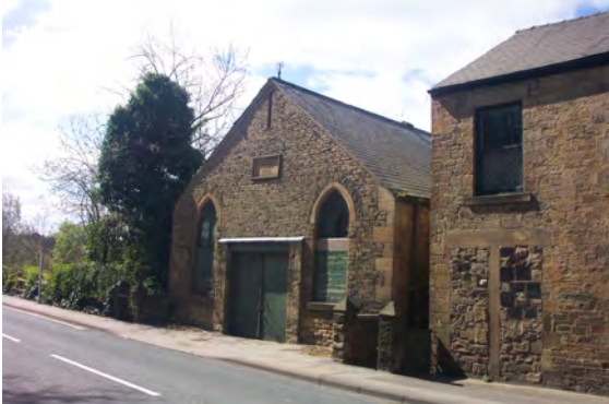
The Assembly Rooms is a prominent, historically significant redundant building in Shotley Bridge
