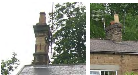
Chimneys are usually constructed of stone, although there are some buff brick examples
