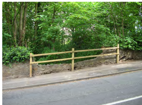
Some boundary walls in the village have deteriorated to an extent that they have collapsed and been replaced with uncharacteristic fencing.
